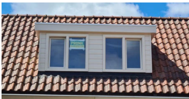
Dakkapel over 2 woningen
